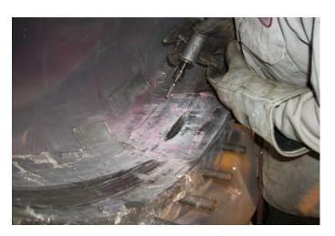
After all areas were protected surrounding the two cracks, the cracks were then excavated. The dye penetration test was repeated many times to make sure the crack was completely excavated.
